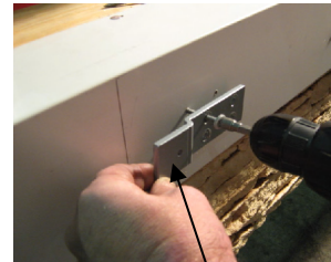
OFFSET FACING LEFT FOR FIRST BRACKET
