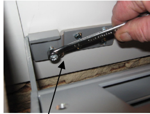
TIGHTEN SET SCREW
