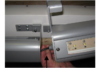
PUSH THE CABLE INTO THE OPEN SIDE OF THE FIXTURE TO THE LEFT
